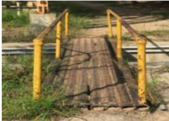
Ramps & supports made from scrap steel
